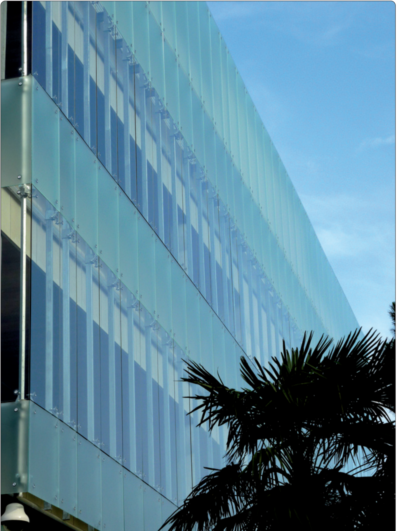
Glasfassade in Zarragoza/Spanien | Glass facade in Zarragoza / Spain
